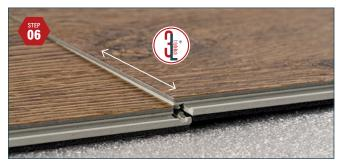
**ENGAGE 3<sup>RD</sup> PLANK ON SHORT SIDE (Part I)** Using the **3L TripleLock** one piece drop-lock system, drop the short side of plank 3 onto the short side of plank 1.
