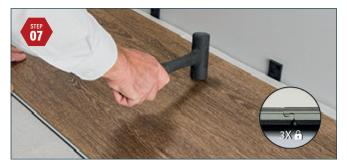
**ENGAGE 3<sup>8D</sup> PLANK ON SHORT SIDE (Part II)** Using a rubber mallet slightly tap the joints on the short side to secure. This ensures 3x locking.
